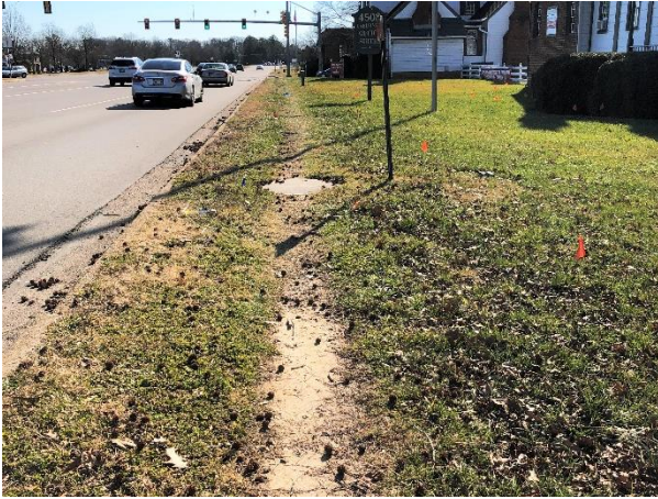
Worn path headed southbound on South Laburnum Avenue approaching Jan Road
