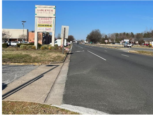
Closely spaced driveways on southbound South Laburnum Avenue between Laburnum Square and US 60 (Williamsburg Road)
