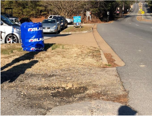
Closely spaced driveways on southbound South Laburnum Avenue north of the Westbound I-64 Ramps
