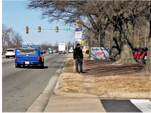
No sidewalk or lighting at GRTC transit stop located just south of Finlay Street
