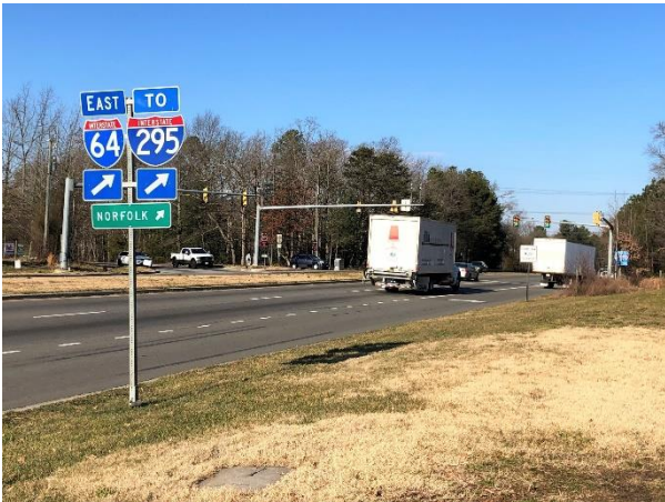
Advanced interstate sign for I-64 East headed northbound on South Laburnum Avenue just south of the Eastbound I-64 Ramps. There is a lack of advanced signing for I-64 West.
