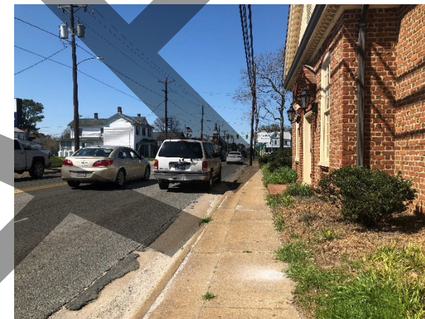
THE FIVE-FOOT WIDE SIDEWALK IS LOCATED IMMEDIATELY BEHIND THE BACK OF CURB WITH NO BUFFER. UTILITY POLES FREQUENTLY REDUCE THE THROUGH WIDTH. BUILDINGS ARE LOCATED WITHIN A FEW FEET OF THE BACK OF SIDEWALK.
