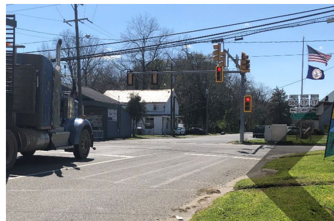
THE WESTBOUND APPROACH OF QUEEN STREET AT US 17 LACKS A DEDICATED LEFT TURN PHASE AND SIGNAGE INDICATING TURNING VEHICLES MUST YIELD TO ONCOMING EASTBOUND VEHICLES.
