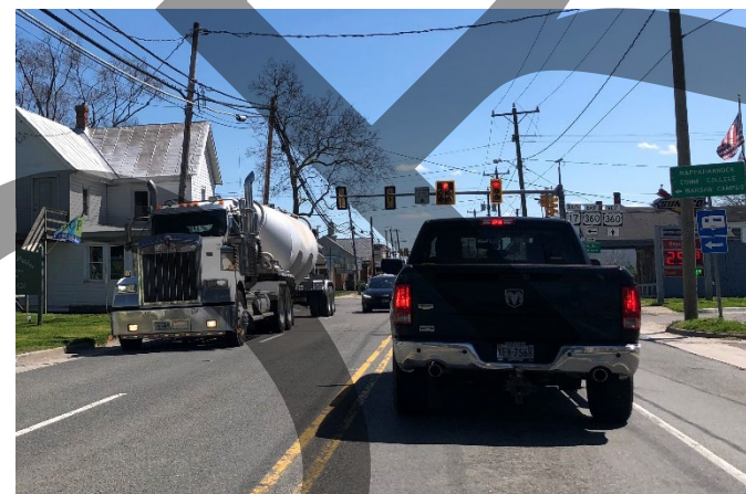
LANES ON US 17 BETWEEN MARSH STREET AND WRIGHT STREET ARE NINE-FOOT WIDE, PROVIDING LITTLE MARGIN FOR ERROR FOR VEHICLES CHANGING LANES. TRUCKS AND OTHER HEAVY VEHICLES COMPRISE 9 PERCENT OF DAILY TRAFFIC VOLUMES.
