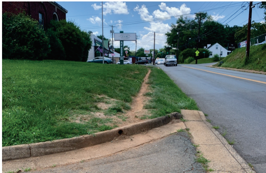
Figure 12. Desire path on the southeast side of East High St
