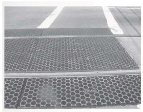
**Figure 16-1.** Installing a rubber surface rather than asphalt on a shared use path is an example of how rail crossings can be improved for pedestrians.
