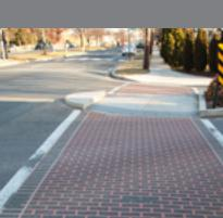
amped asphalt crosswalk. ocation: N Brookside Drive and Washington vd., Arlington, VA
