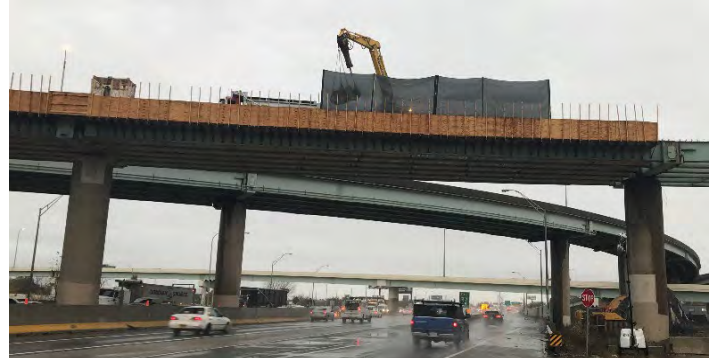
Demolition over I-95 in Philadelphia Betsy Ross Bridge
